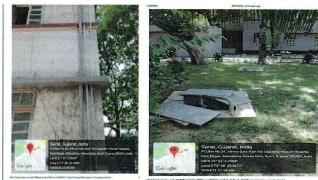
Figure: rain water harvesting collection pipe and tank
